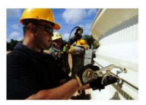
The roof panels assembly is then fixed to super structure either in Steel or RCC by Anchor fastener or nut and bolts as per design.
