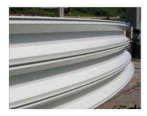
A set of three panels are assembled and mechanically seamed together at ground level and using specially designed lifting tackles are hosted in to position by cranes.
